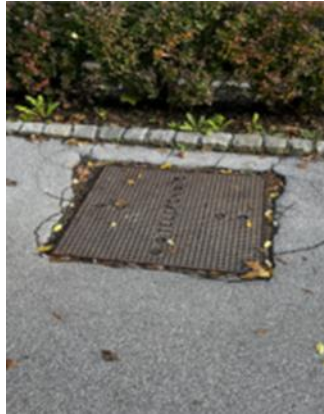
Picture 2: Utility shaft.
