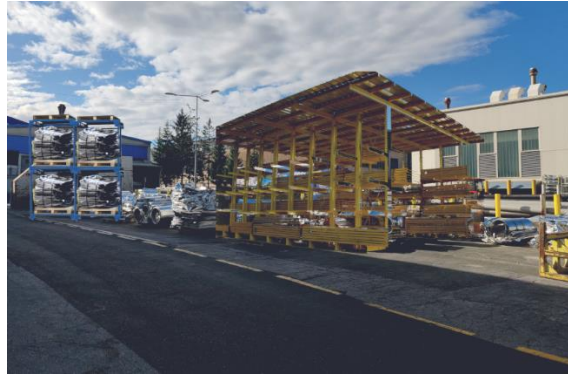
Figure 68: Installation of pallet racks and cantilever racks Source: Own
